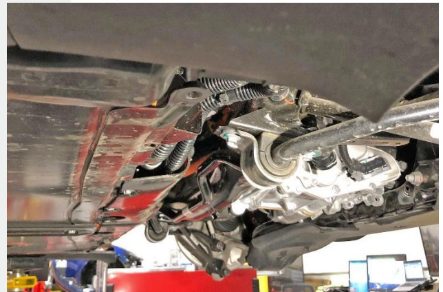
✗ Figure 4 – Mid aero shield panel missing
